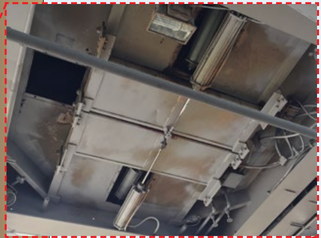
SHOWN: 5 x 24 safety gate cylinders, 6 x 20 discharge cylinders
